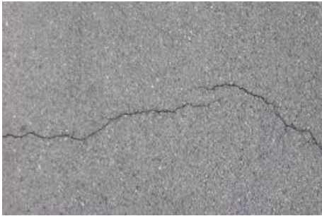
Figure 1. Road Crack
